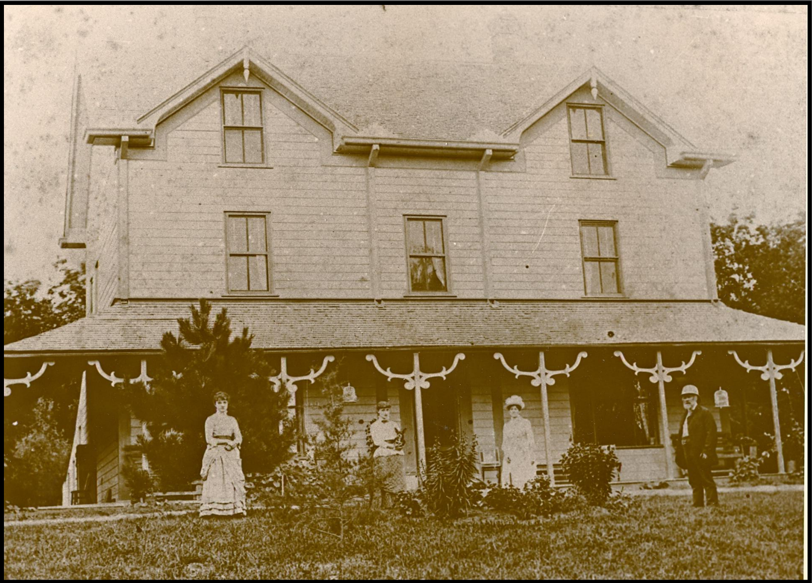
Joseph Ramsdale Home, built in 1878. It later Became Hazelmere Resort, located off of Albion Ave. Between Lake View & Alton Street St.
