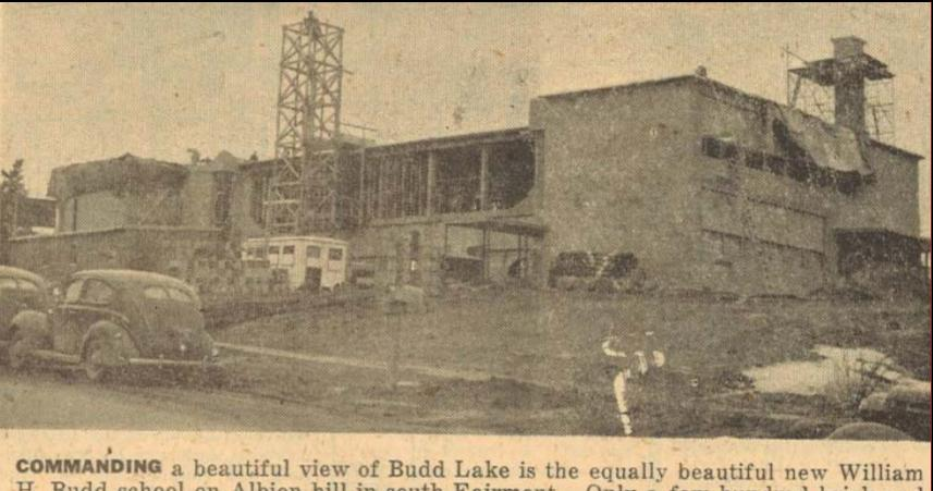
H. Budd school on Albion hill in south Fairmont. Only a few hundred brick and glass block are still to be installed to complete the shell of this building. Mud is slowing this operation. The auditorium is the wing at the far left, and the balance of the building is classrooms.—Guckeen Photo-Engraving.
