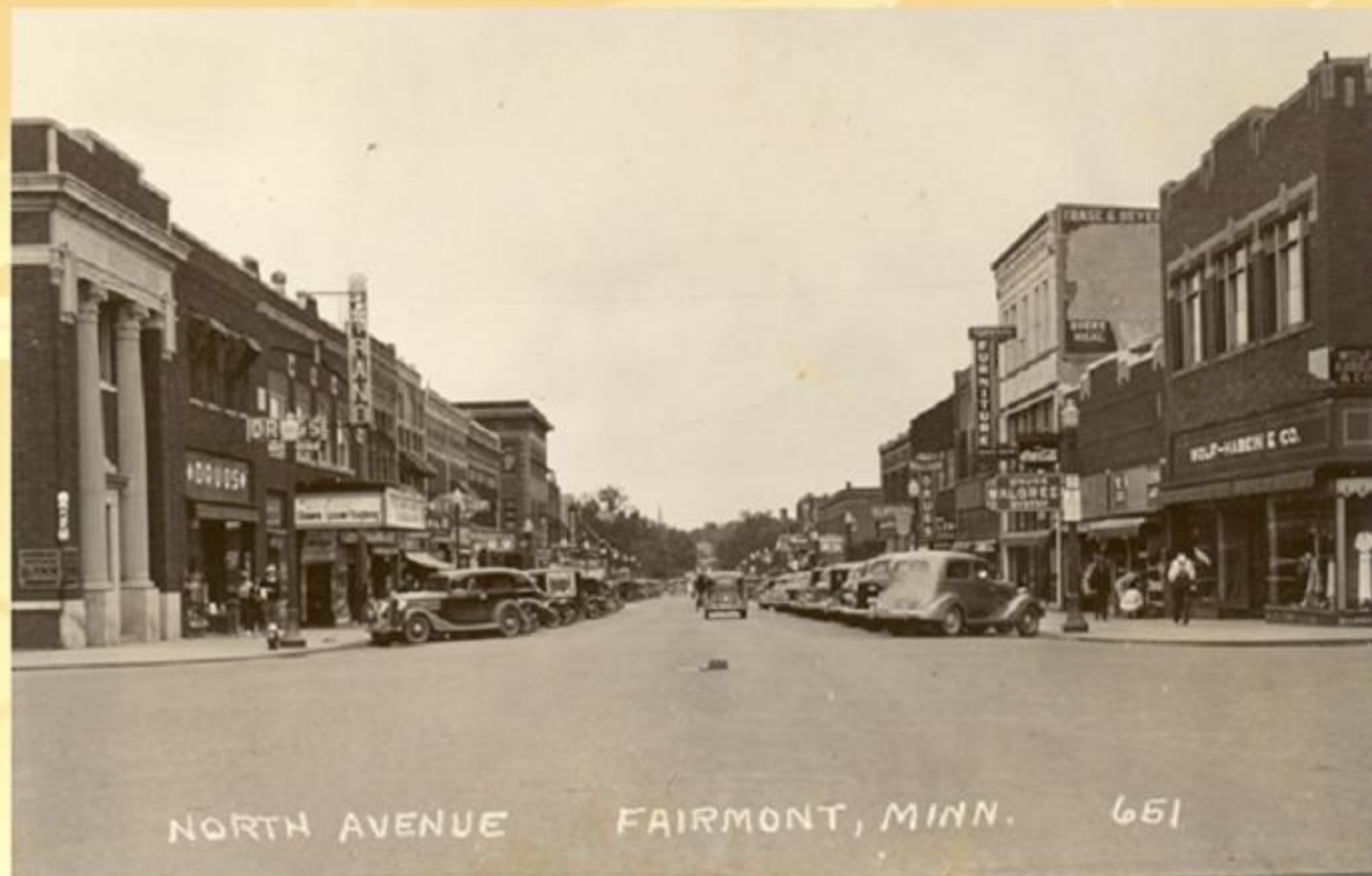
100 Block North North Avenue
