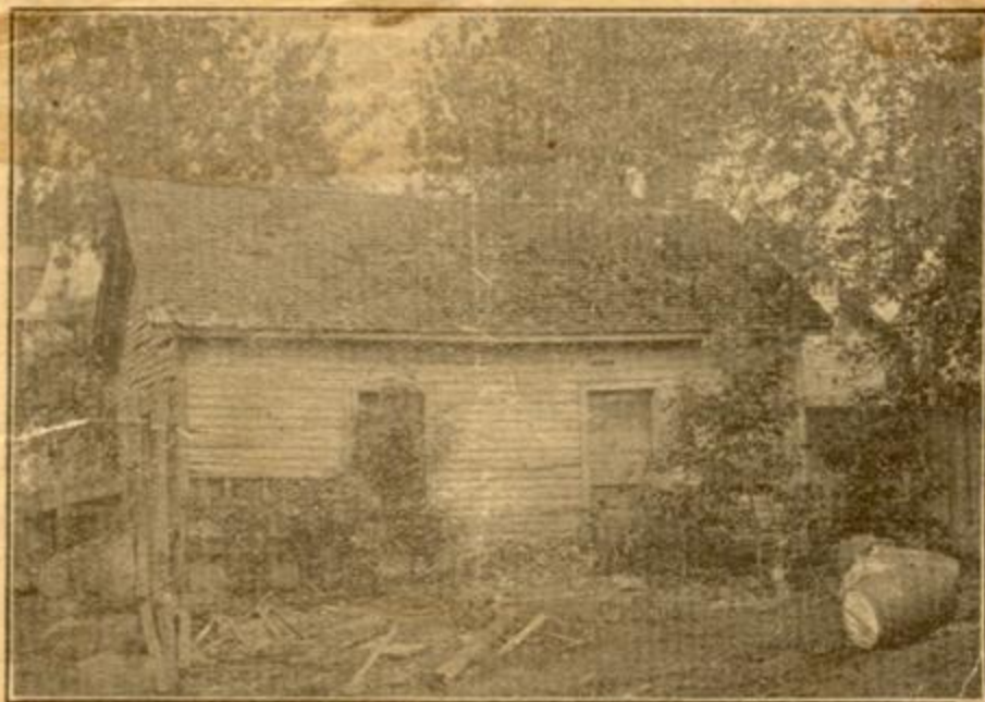
MARTIN COUNTY'S PIONEER COURT HOUSE
